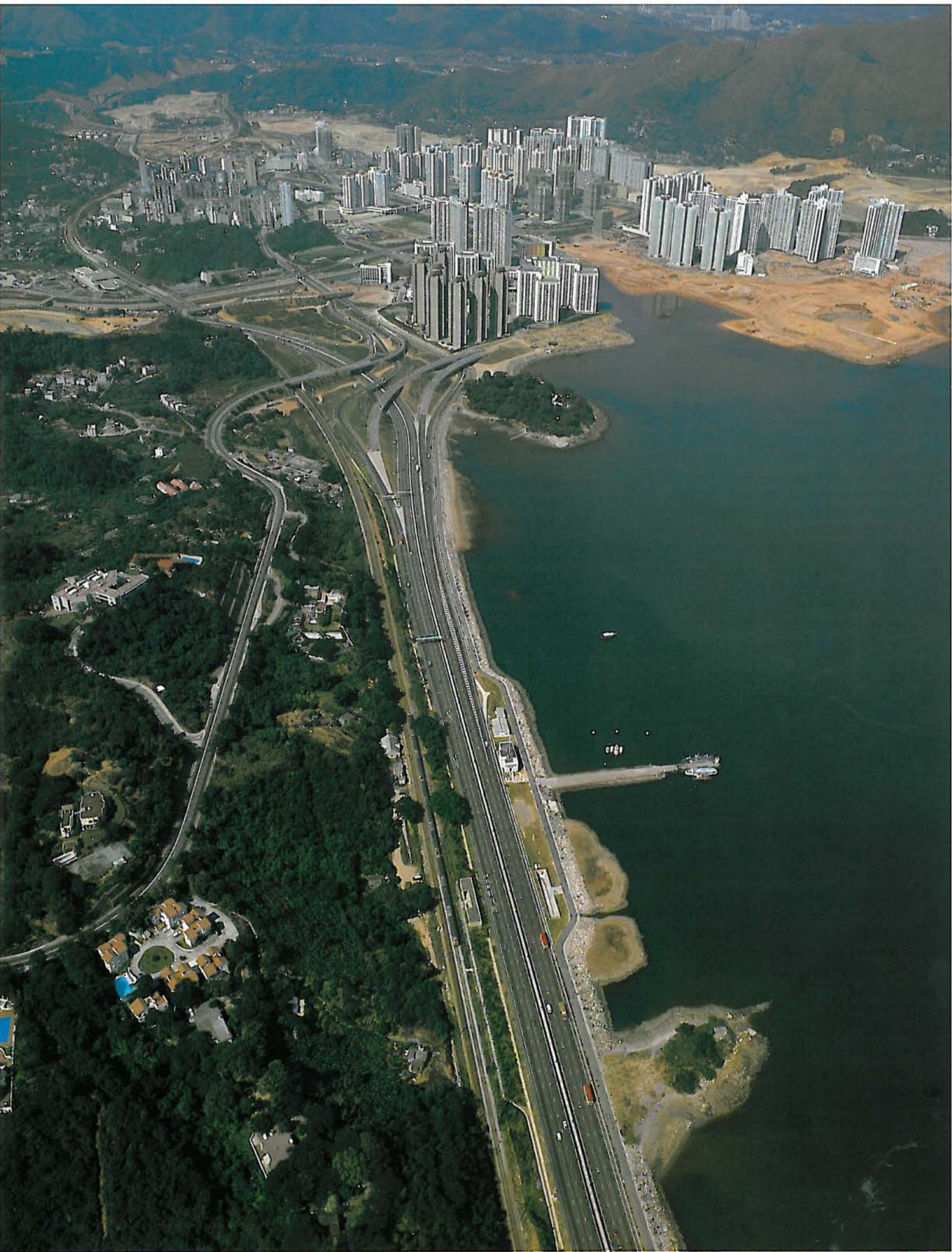
Taipo, another of Hong Kong's satellite towns in the New Territories, shows the scars of recent reclamations. The section of the New Territories circular highway linking Taipo with Shatin is also shown.
