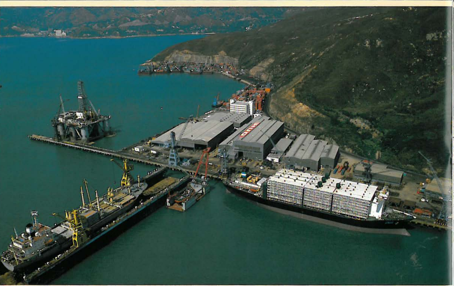
(Top) Hong Kong's new Eastern Approaches Harbour Tunnel, now under construction, will provide road and rail connection between Hong Kong Island and Eastern Kowloon. Photo shows the northern end of the tunnel at Cha Kwo Ling. (Bottom) Tsing Yi Island, where most of Hong Kong's ship repairing and conversion yards are located. Oil rigs and platforms are also constructed and modified. (上) 香港現正興建新的東區過海隧道，以道路及鐵路連接港島及東九龍，圖中所見為位於茶果嶺的隧道北口。(下) 香港有很多船隻修理及改裝工場設於青衣島，島上亦興建及改進鑽油設備及鑽油台。
