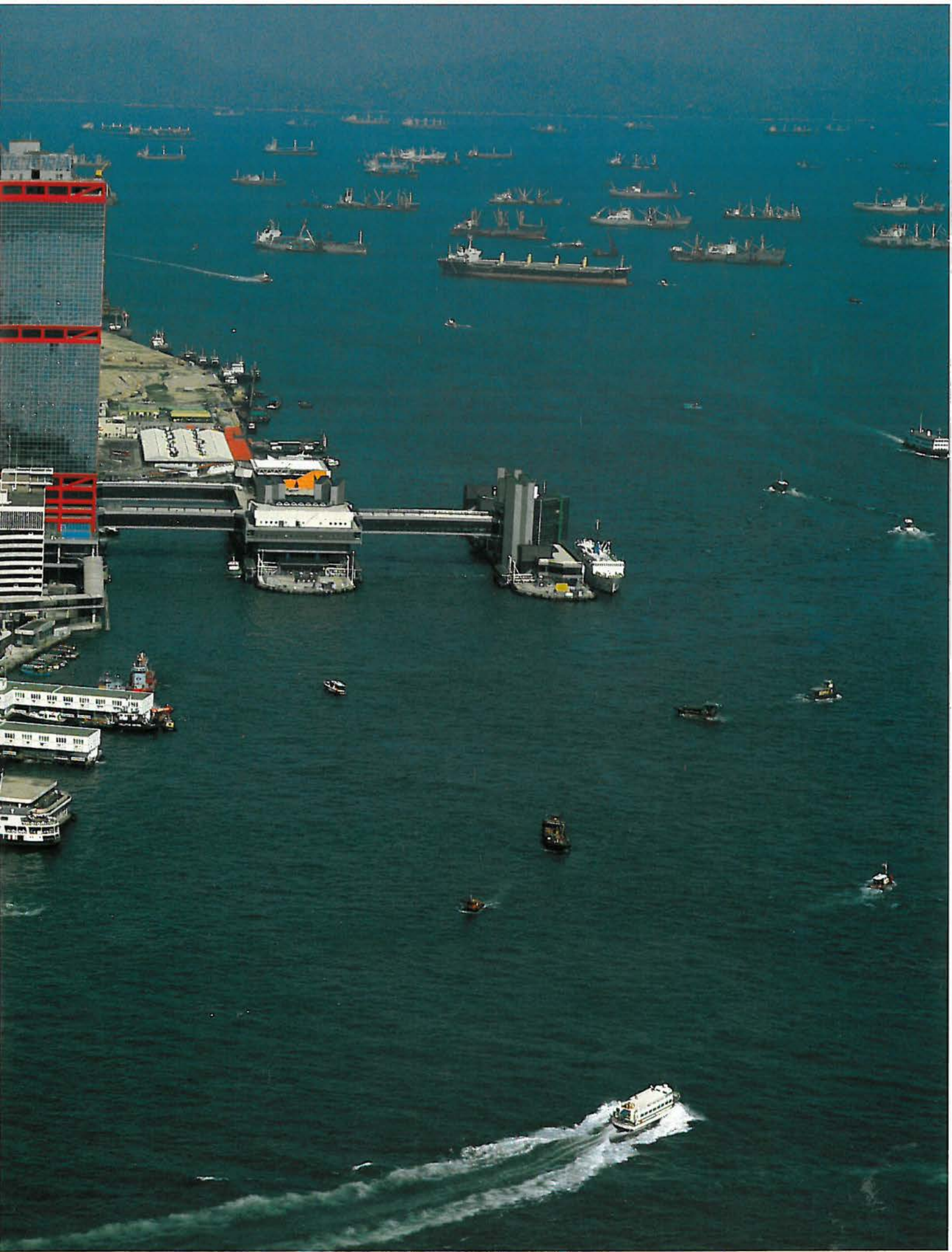
High-rise buildings, many still under construction, crowd the slopes leading down to the Western District waterfront on Hong Kong Island. Hong Kong's maritime character is amply demonstrated by the merchant ships at anchor. 高樓大廈緊密擁聚，一直向港島西區海傍伸延開去，其中很多仍在施工。海港商船滿佈，充分表現香港的海運地位。
