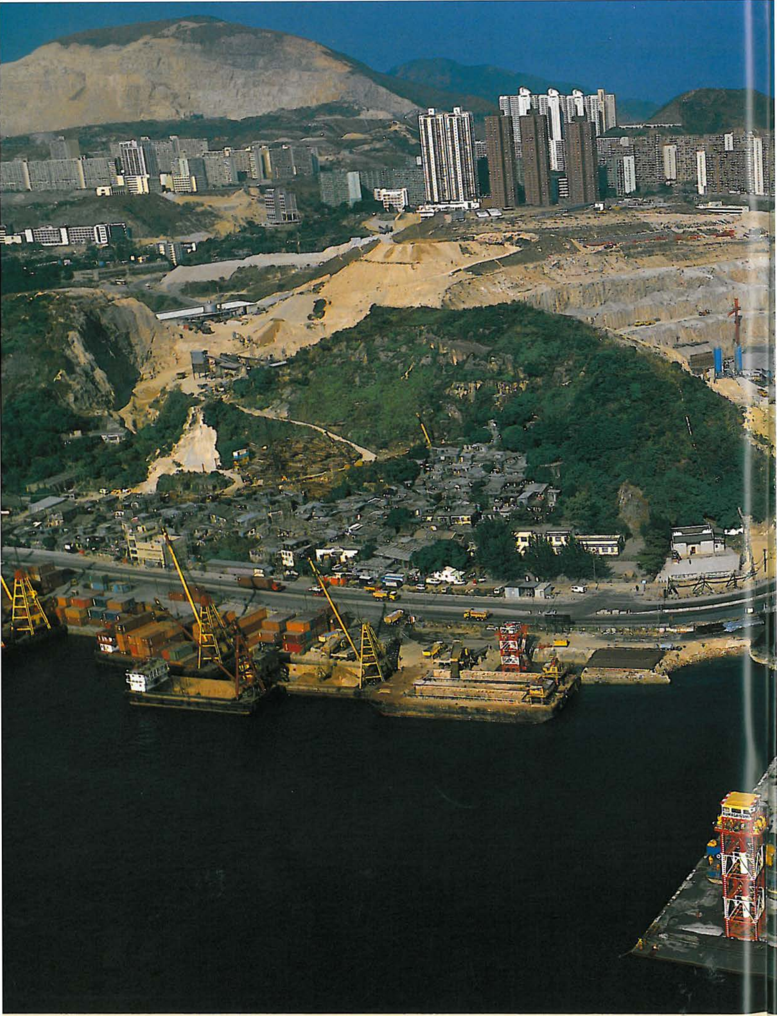
Excavation scars Cha Kwo Ling as Hong Kong builds its Eastern Harbour Tunnel, that next year will more than double cross-harbour traffic capacity.
