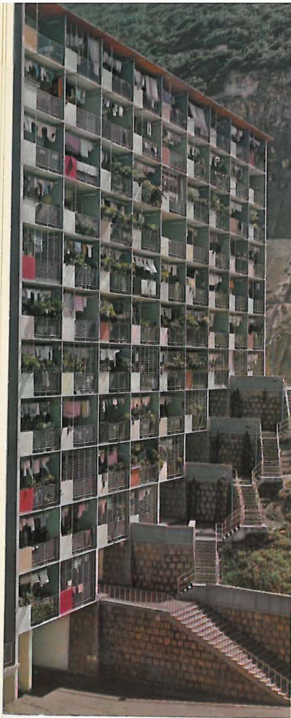
Building up hillside
