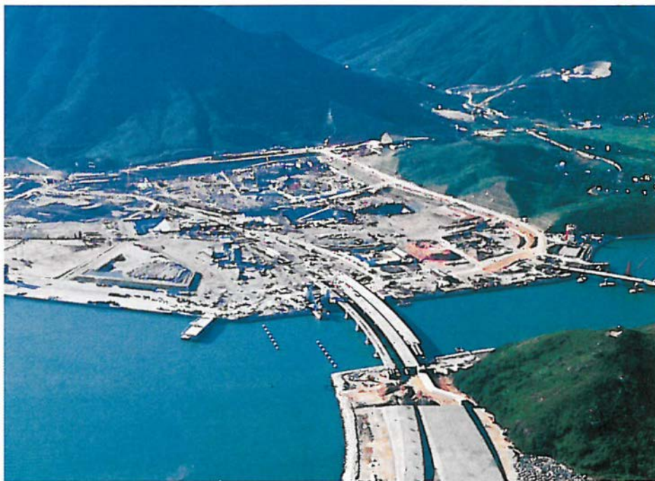
Update on Chek Lap Kok progress and the road and rail bridges linking the new airport to Tung Chung new town on North Lantau.
