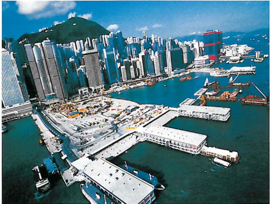
New ferry piers on the Central Reclamation.
