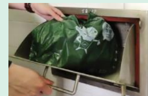
The inlet of the refuse chute on individual floor
