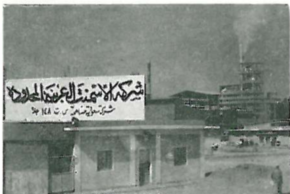
An industrial area in Saudi Arabia
